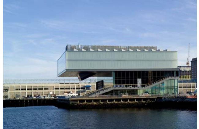
West view The Institute of Contemporary Art, Boston Diller Scofidio + Renfro Architects Credit: Peter Vanderwarker
